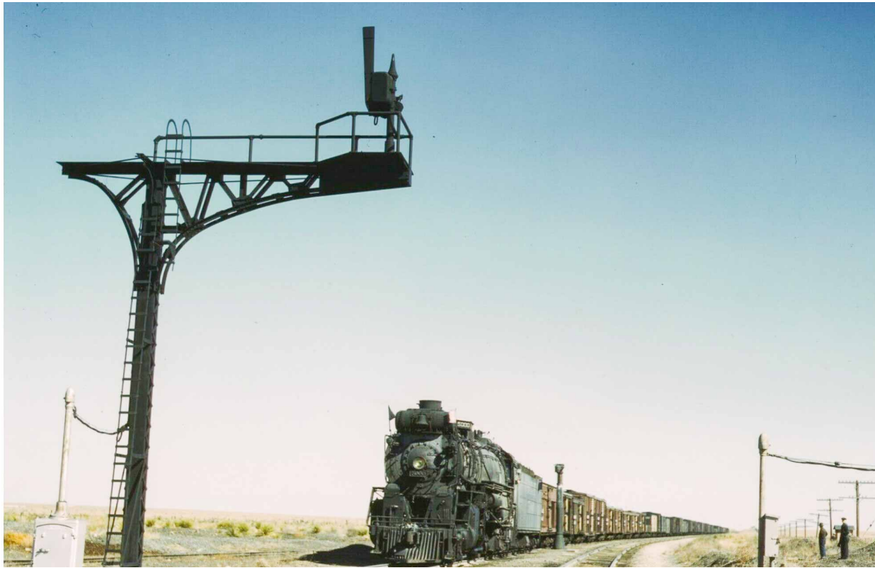
JACK DELANO'S PHOTO IN RICARDO, 1943. THE "MADAM QUEEN" (LOCOMOTIVE 5000), IS SITTING IN THE SIDING AT THE WEST SWITCH. NOTE THE WATER STANDPIPE NEXT TO THE TENDER OF THE LOCOMOTIVE.
